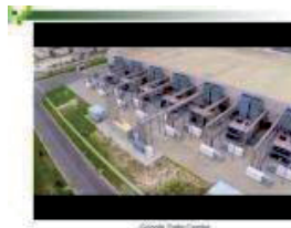
Google Data Center
